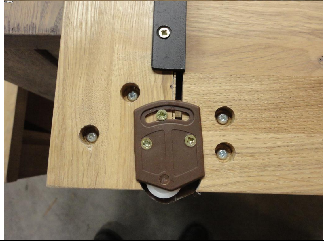
Adjustable wheel for sliding door. By the use of this it can open and close more easy
